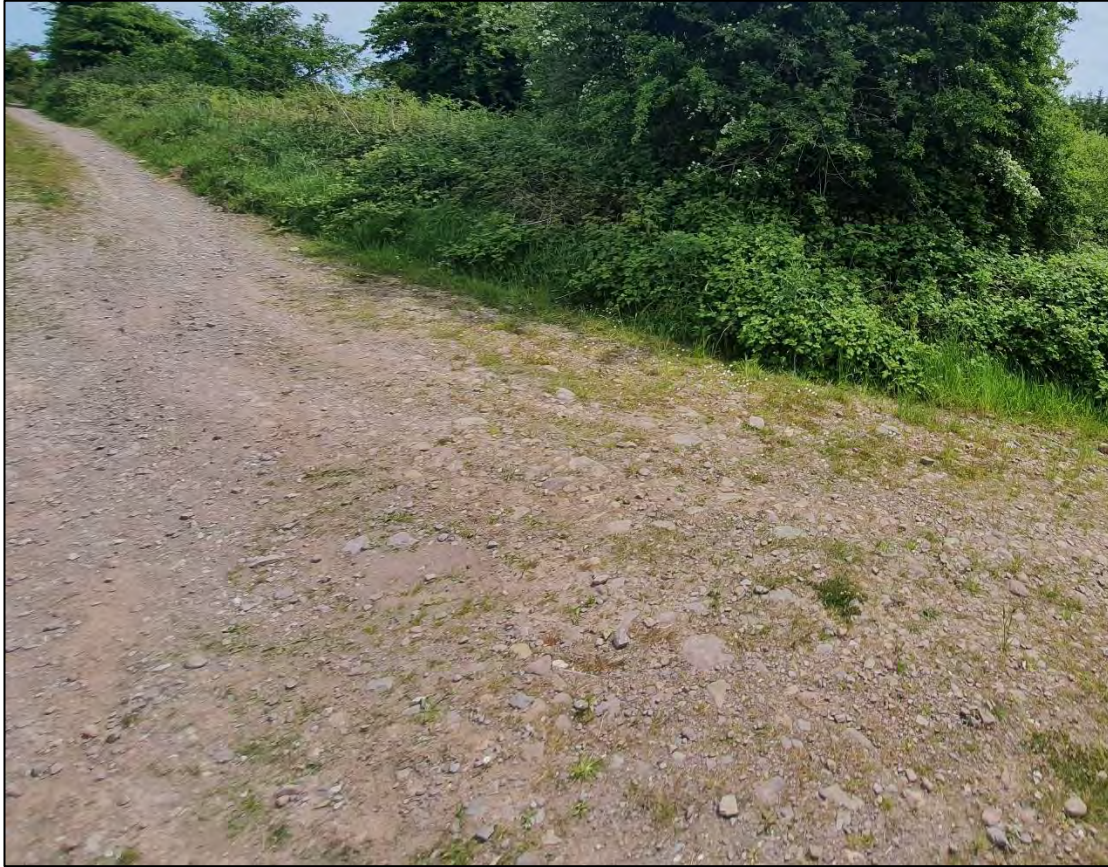
Plate 4-10 Example of existing on site access roads (BL3)
