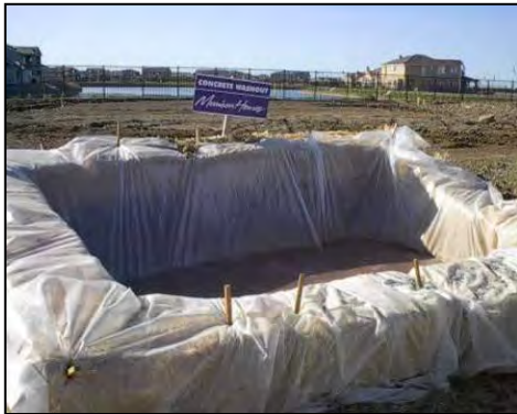
Plate 4-1 Concrete washout area
