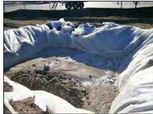
Plate 4-2 Concrete washout area
