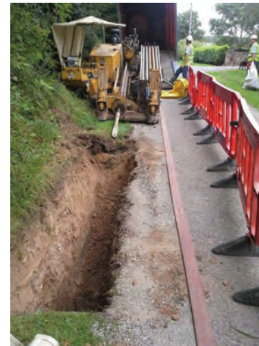
Typical Drilling Rig & Launch Pit
