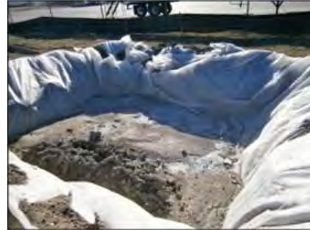
Plate 4-4 Concrete washout area
