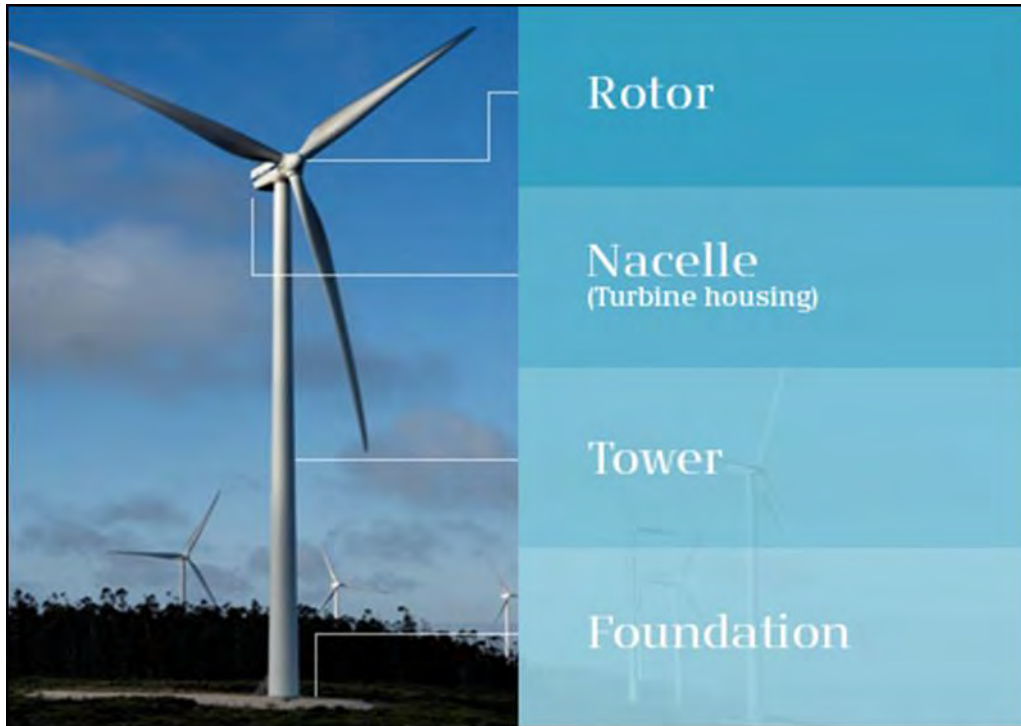
Plate 4-1 Wind turbine components
