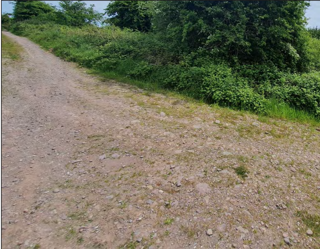
Plate 7-10 Example of existing onsite access roads
