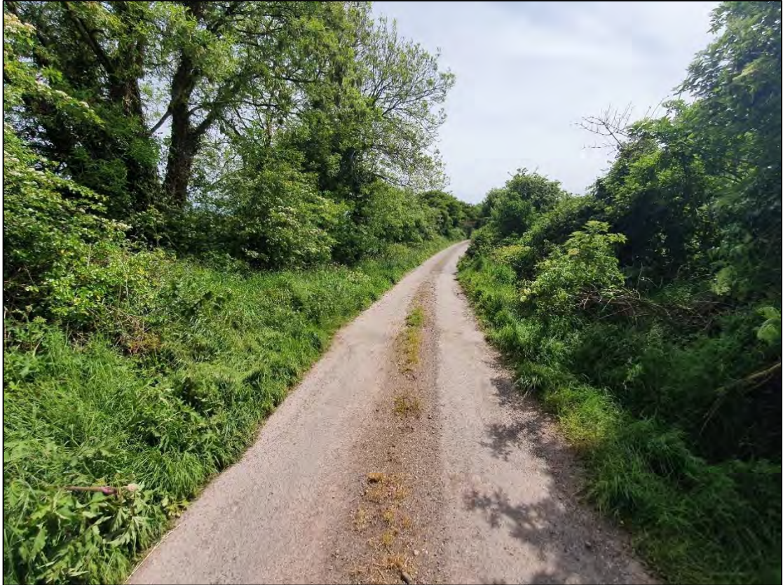
Plate 7-17 Local road along which the turbine collector cable route will be located for part of the route.
