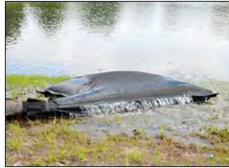
Plate 4-6 Silt bag with water being pumped through
