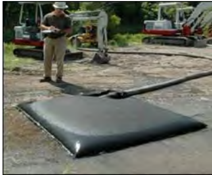
Plate 4-5 Silt Bag under inspection
