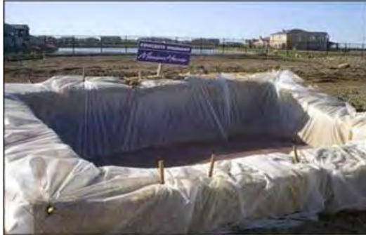
Plate 4-3 Concrete washout area
