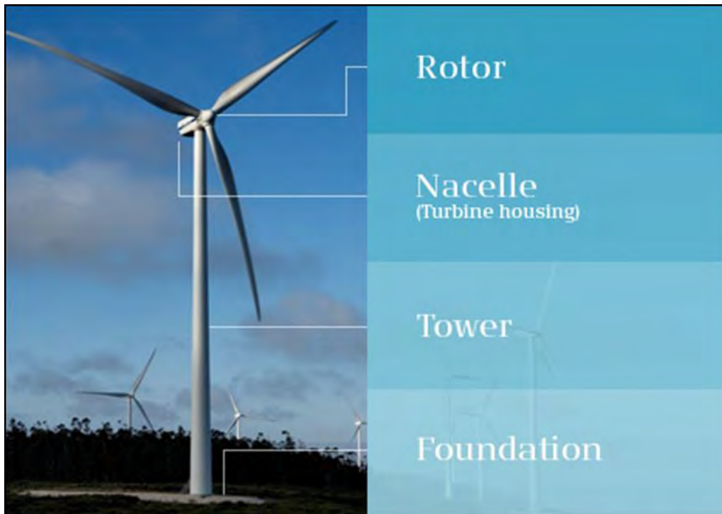
Plate 4-1 Wind turbine components
