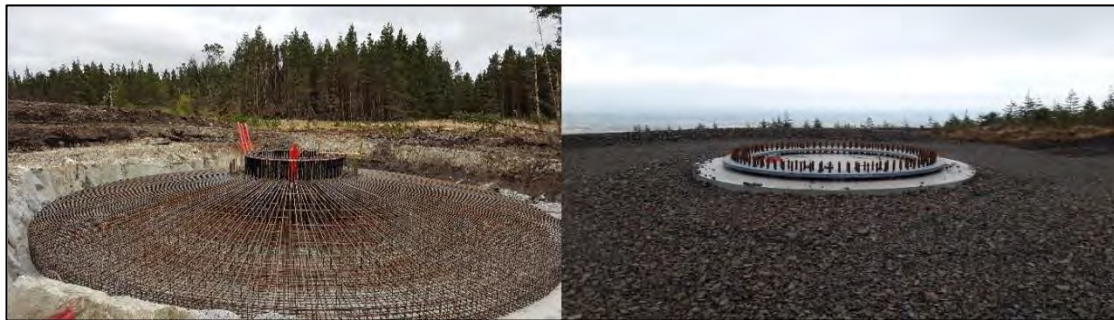
Plate 4-2 Turbine 'Anchor Cage' (left) and finished turbine base (right)
