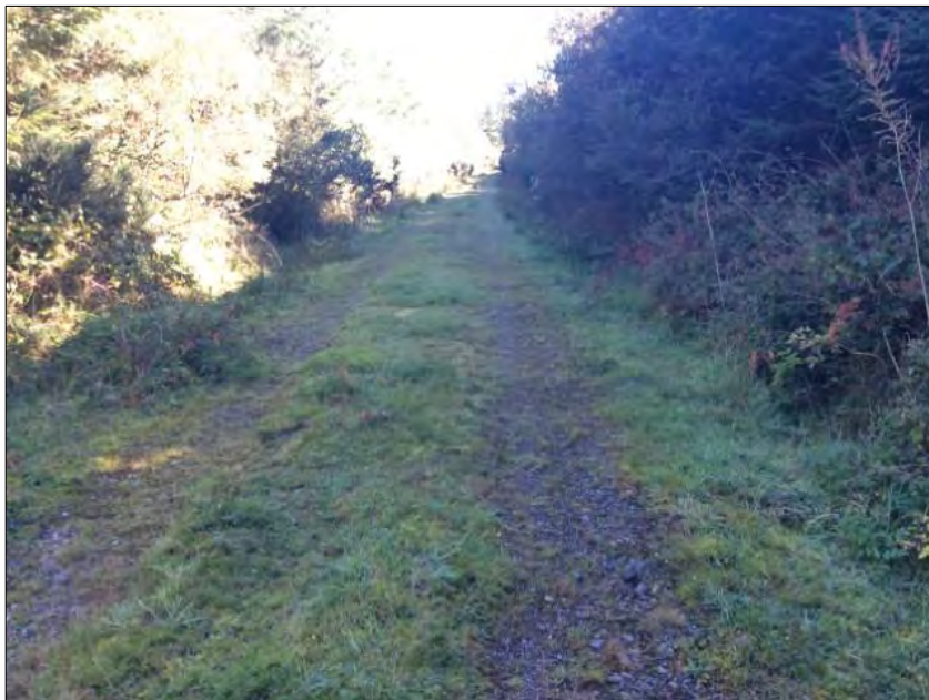
Plate 14.14: Existing road due for upgrade to the E of Turbine 2 looking east.
