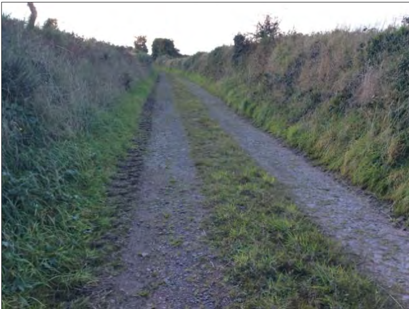
Plate 14.26: Existing road south of T7, looking west.
