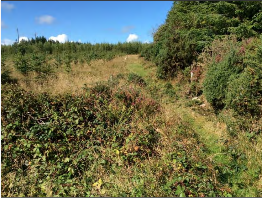
Plate 14.50: Route of proposed road to T17 along break in forestry, looking NW.
