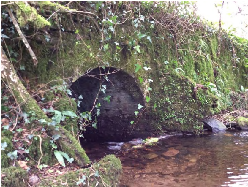
Plate 14.64: Same as above showing single arch stone bridge.
