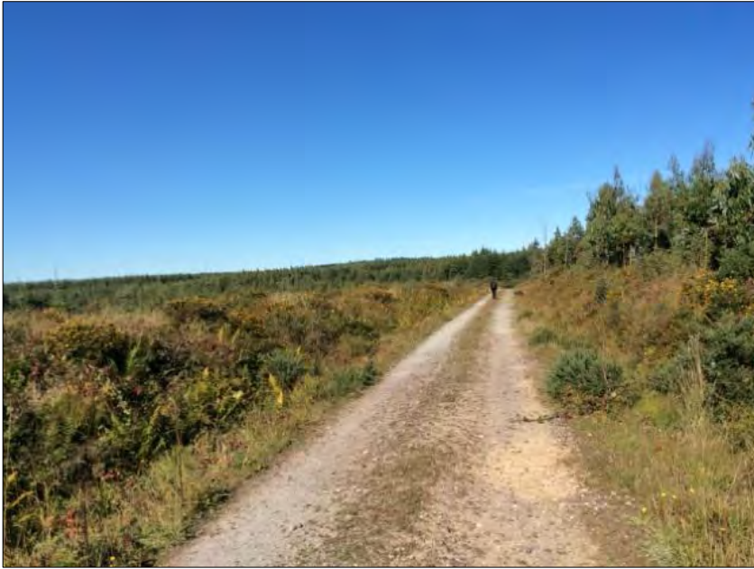
Plate 14.5: Existing road due for upgrade to the south of T1, looking NW.
