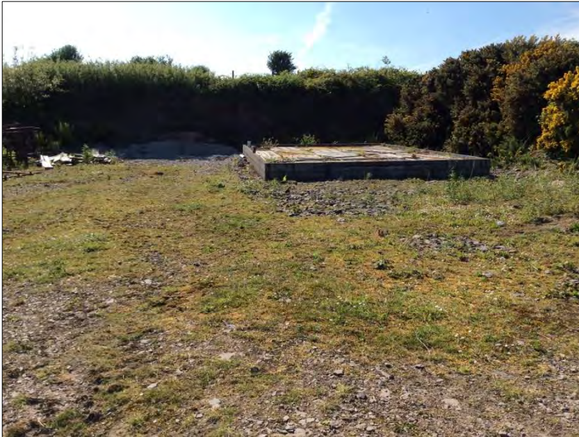
Plate 14.52: Met mast compound looking NW.
