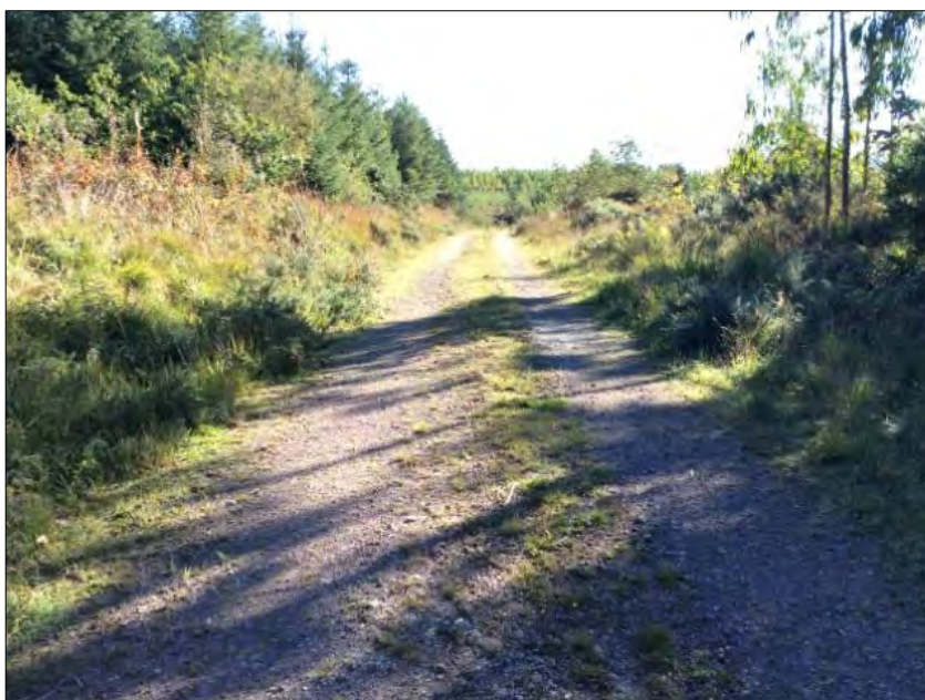
Plate 14.2: Continuation of existing access road looking E, in the direction of T1.
