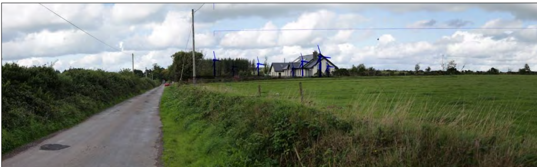
Plate 12-20 Wireframe overlaid on photographs taken at AV6 looking north towards the proposed western turbines
