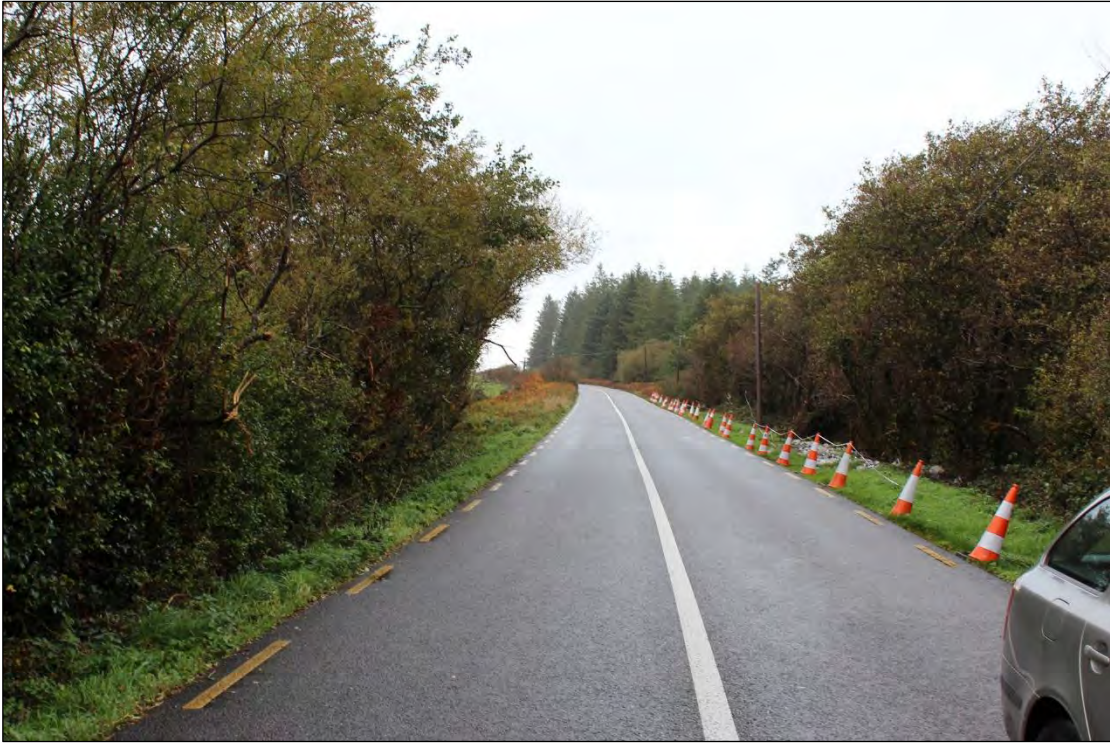
Plate 12-25 View looking northwards taken at location RSA1 shown on Figure 12-15 classed as ‘intermittent’ in the Route Screening Assessment
